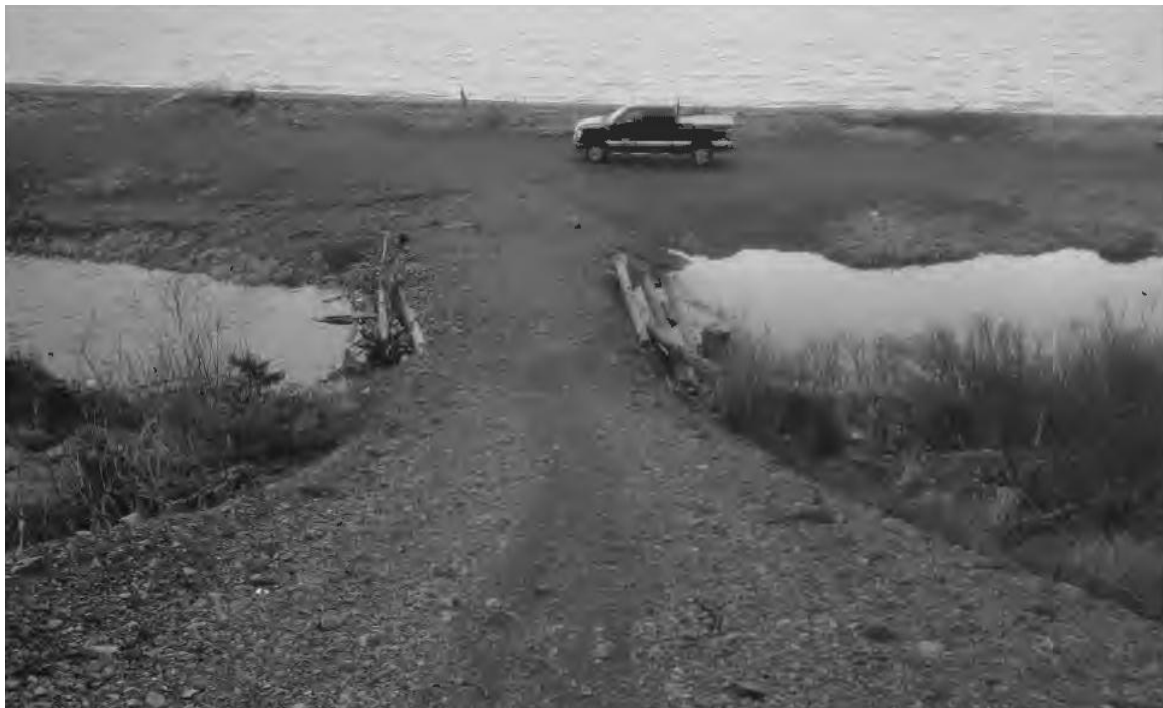
Image 2: Newly Constructed Causeway, 2017, with Enforcement Vehicle
