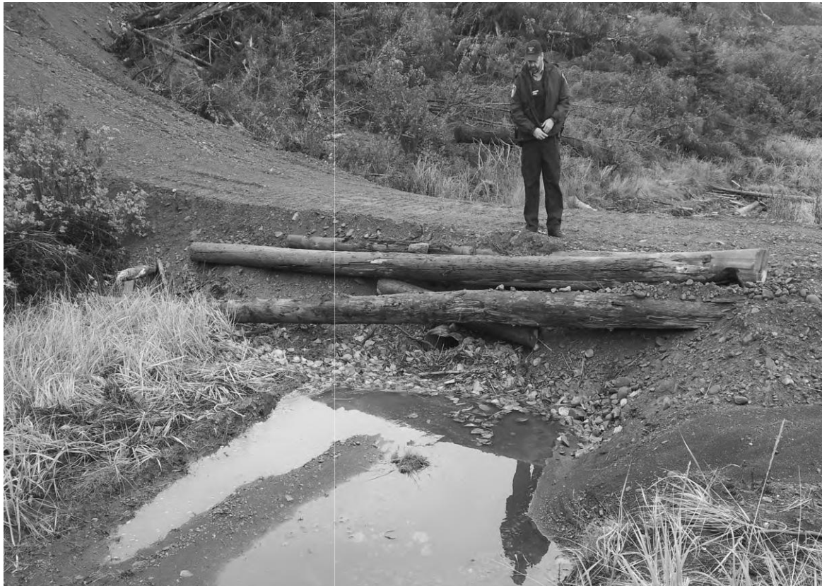
Image 1; Newly Constructed Causeway, 2017, with Enforcement Officer
