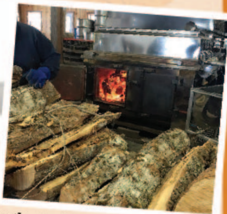
to the boiler ...
