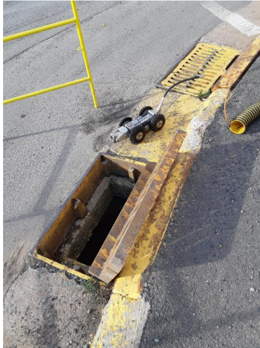
Figure 3 Remote Controlled Camera Preparing to enter catch basin
