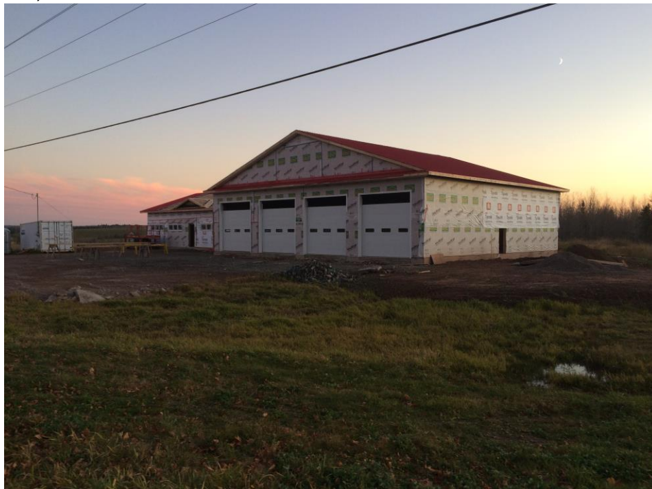
Figure 4 Shinimicas Fire Hall Nov 8, 2021
