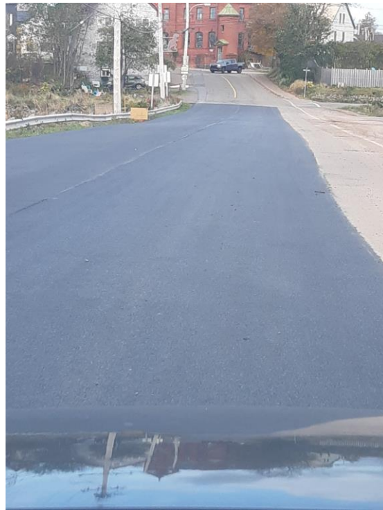
Figure 1 Asphalt Overlay on Two Island Rd. Parrsboro
