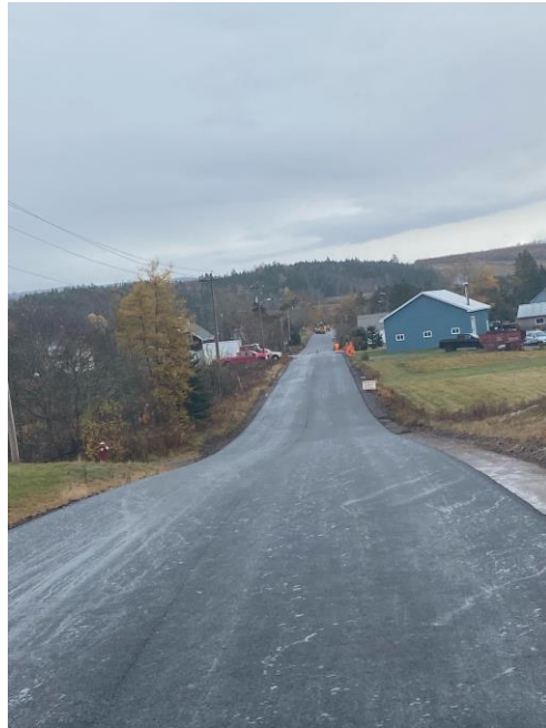
Figure 2 Asphalt Overlay on Farrell Rd. Parrsboro
