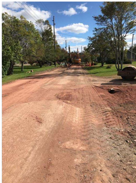
Figure 1 Layton St. Waterline Replacement
