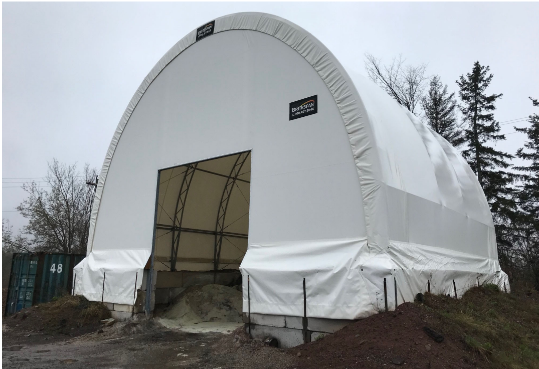
Similar 36' x 32' structure in Oxford NS
